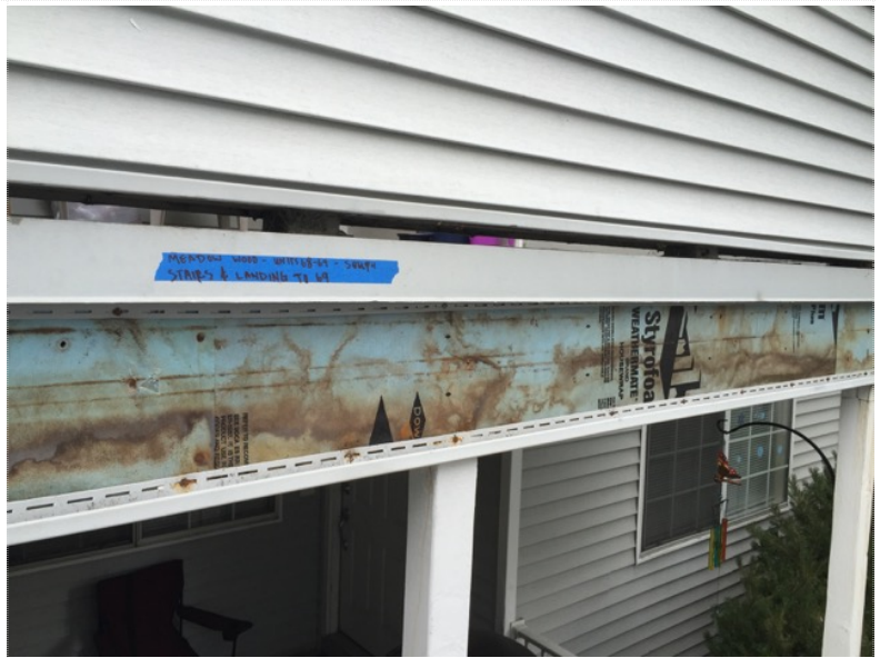
1.131 Exploratory Opening #15 Unit 68 - 69 - Access Landing
