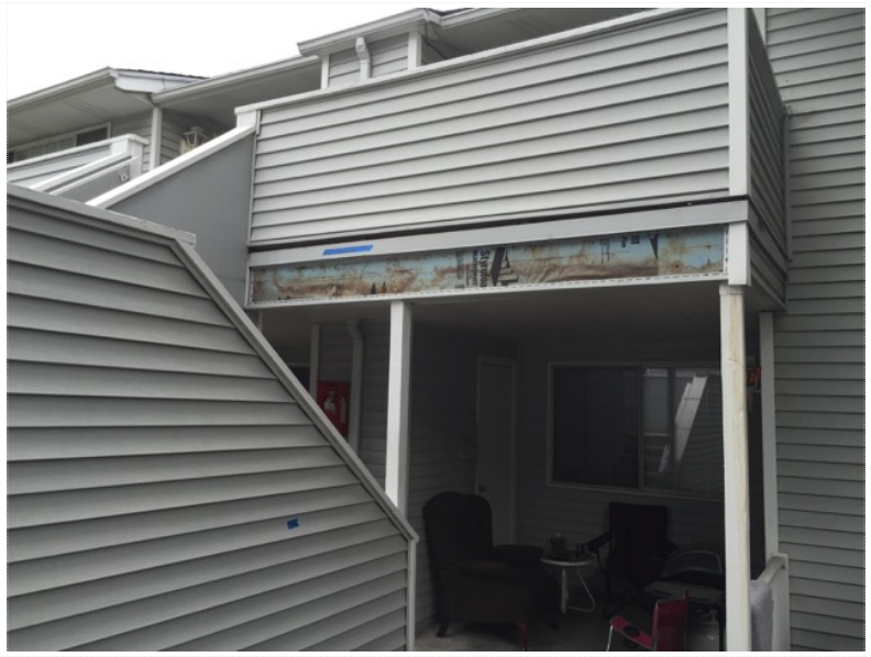
1.130 Exploratory Opening #15 Unit 68 - 69 - Access Landing
